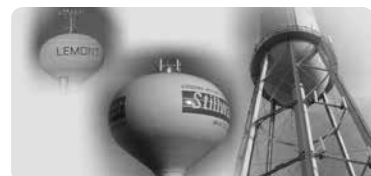
Water Tower Applications
